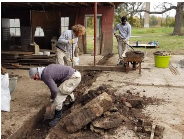
Digging out debris to prepare for cement footing 10/25/19
